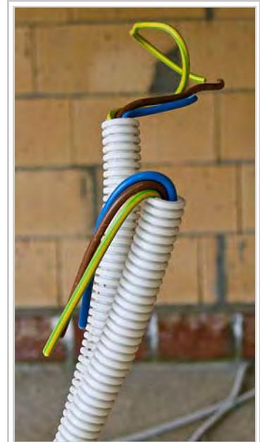
Colour-coded wires in a flexible plastic electrical conduit found commonly in modern European houses
