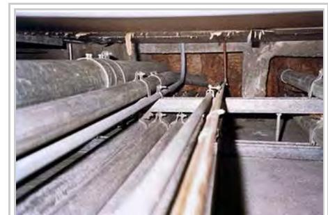
Electrical conduit risers, seen inside fire-resistance rated shaft, as seen entering bottom of a firestop. The firestop is made of firestop mortar on top, rockwool on the bottom. Raceways are used to protect cables from damage.
