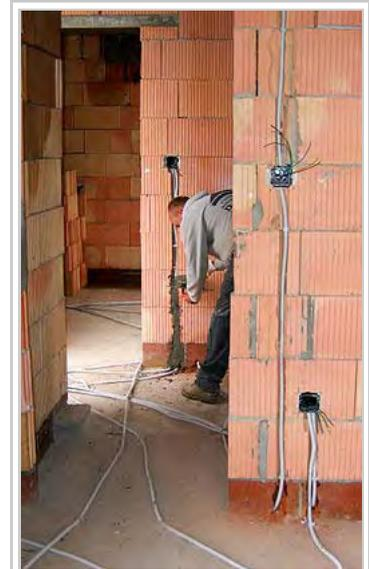
Installing electrical wiring by "chasing" grooves into the masonry structure of the walls of a building
