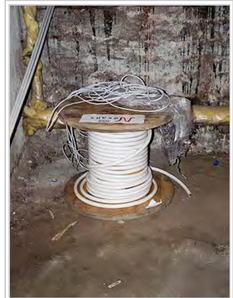
5 core PVC insulated copper cable
