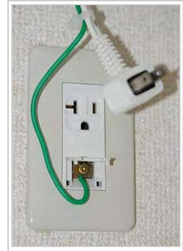
Japanese socket with earth post and earth connector, for an air conditioner
