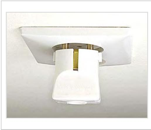
CEE 7/4 plug partially inserted into CEE 7/1 socket: the pins are exposed and there is no connection for the plug's earthing contacts
