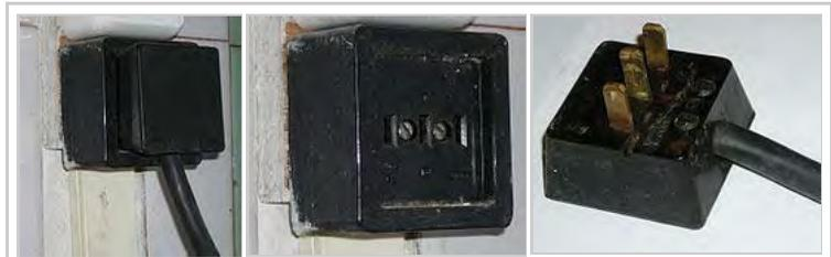
Russian stove connectors rated 250 V 25 A AC. Left: plug and socket. Center: Socket. Right: Plug.
