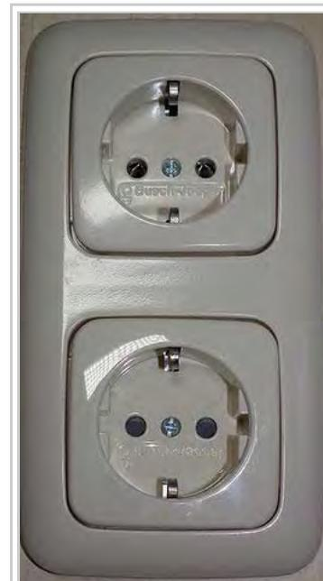
Two Schuko (CEE 7-3) socket-outlets manufactured by Busch-Jaeger Elektro GmbH, the lower has protective shutters, the upper does not.
