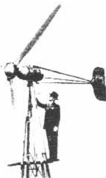
Marcellus Jacobs stands on tower holding his 3-kilowatt wind electric plant in this vintage 1940s portrait.
