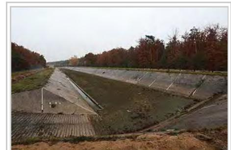
Slow "artificial" filtration (a variation of bank filtration) to the ground, Water purification plant Káraný, Czech Republic
