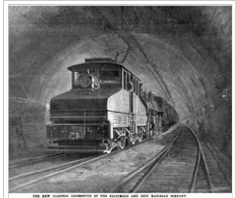
Electric locomotive of the Baltimore Belt Line, 1895: The steam locomotive was not detached for passage through the tunnel. The overhead conductor was a \cap section bar at the highest point in the roof, so a flexible, flat pantograph was used
