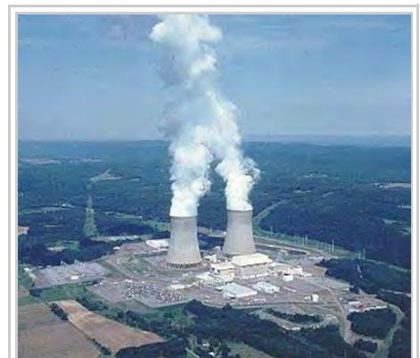
A power station's cooling tower produces clouds from the condensing water vapor due to evaporated cooling water.
