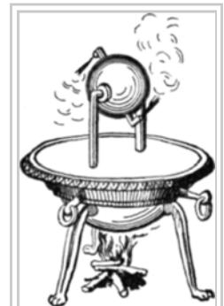
An aeolipile rotates due to the steam escaping from the arms. No practical use was made of this effect.
