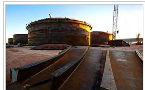
Construction of the Salt Tanks which provide efficient thermal energy storage<sup>[100]</sup> so that output can be provided after the sun goes down, and output can be scheduled to meet demand requirements.<sup>[101]</sup> The 280 MW Solana Generating Station is designed to provide six hours of energy storage. This allows the plant to generate about 38 percent of its rated capacity over the course of a year.<sup>[102]</sup>
