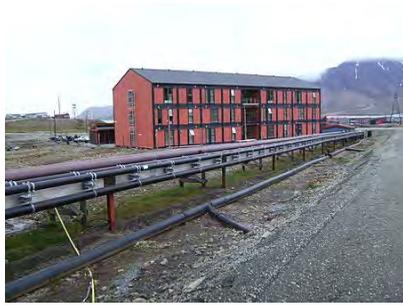
Above-ground utility lines in a permafrost zone avoid thawing of ground.
