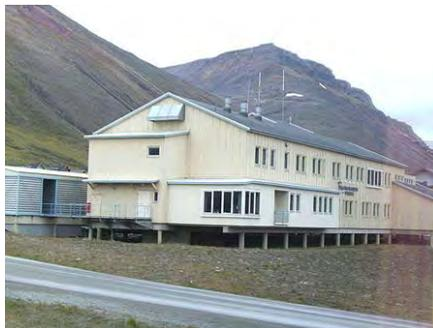
Modern buildings in permafrost zones may be built on piles to avoid permafrost-thaw foundation failure from the heat of the building.
