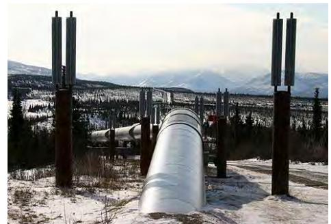
Heat pipes in vertical supports maintain a frozen bulb around portions of the Trans-Alaska Pipeline that are at risk of thawing.
