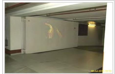
Large fire door, sealing a fallout and air raid shelter inside the basement parking garage of a hotel in Germany.
