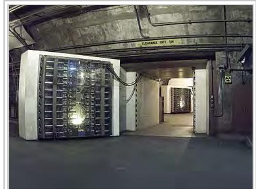
The 25-ton blast door in the Cheyenne Mountain nuclear bunker is the main entrance to another blast door (background) beyond which the side tunnel branches into access tunnels to the main chambers.
