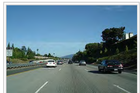
Concrete roadway in San Jose, California
