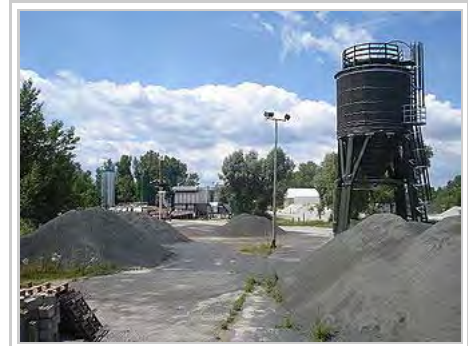
An asphalt mixing plant for hot aggregate
