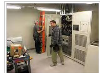
A large datacenter-scale UPS being installed by electricians
