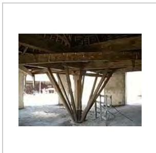
Horse shaft fixed to one of four long beams, all braced to each other with stretchers, and each fixed to the side of the top of the main axle.
