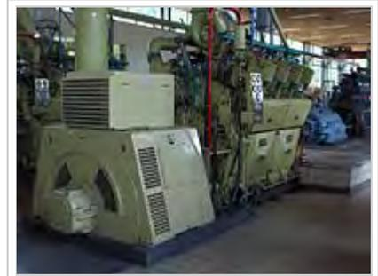
Emergency power electric generator in a drinking water pumping station. Brons engine with N.V.Heemaf generator.
