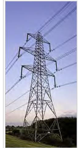
Two-circuit, single-voltage power transmission line; "Bundled" 4-ways
