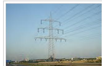
Four-circuit, two-voltage power transmission line; "Bundled" 2-ways
