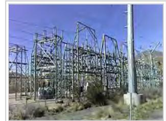
A transmission substation decreases the voltage of incoming electricity, allowing it to connect from long distance high voltage transmission, to local lower voltage distribution. It also reroutes power to other transmission lines that serve local markets. This is the PacifiCorp Hale Substation, Orem, Utah, USA
