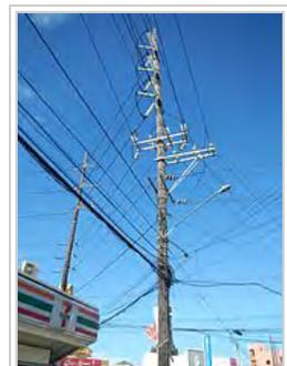
A 115 kV subtransmission line in the Philippines, along with 20 kV distribution lines and a street light, all mounted in a wood subtransmission pole
