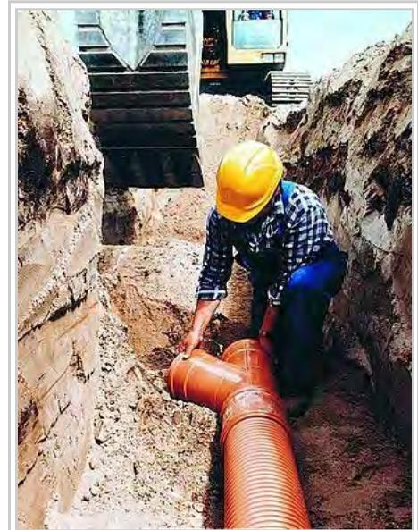
PVC is used extensively in sewage pipe due to its low cost, chemical resistance and ease of jointing
