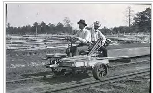
3-wheeled velocipede or handcar on a railroad track. It is operated by hand.
