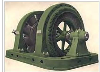
A synchronous motor-generator set for AC to DC conversion, circa 1909
