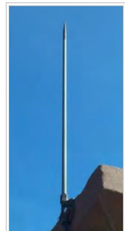
An example of a standard, pointed-tip, air terminal.
