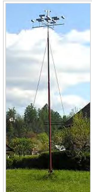
"Machina meteorologica" invented by Diviš worked like a lightning rod
