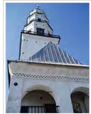
Nevyansk Tower in Russia crowned with a metallic rod grounded through a complex system of rebars (some are seen at the basement)
