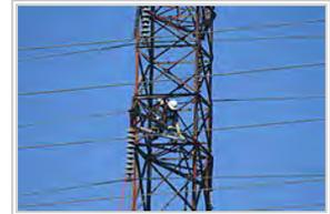
Powerline worker performs maintenance of a lightning arrester on an electrical transmission tower in New Brunswick, Canada.
