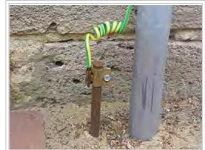
A typical earthing electrode (*left of gray pipe*), consisting of a conductive rod driven into the ground, at a home in Australia. Most electrical codes specify that the insulation on protective earthing conductors must be a distinctive color (or color combination) not used for any other purpose.
