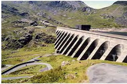
Pumped-storage hydroelectricity – the upper reservoir (Llyn Stwlan) and dam of the Ffestiniog Pumped Storage Scheme in north Wales. The lower power station has four water turbines which generate 360 megawatts (480,000 hp) of electricity within 60 seconds of the need arising.
