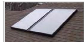
Flat-plate solar thermal collector, viewed from roof-level
