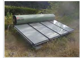
Direct-gain solar heater panels with integrated storage tank
