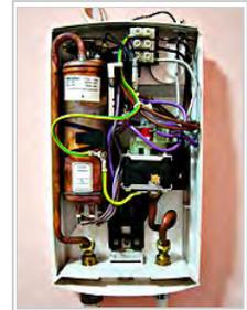
The inside of a hydraulically operated two-stage tankless heater, heated by 3-phase electric power. The copper tank contains heating elements with 18kW maximum power.
