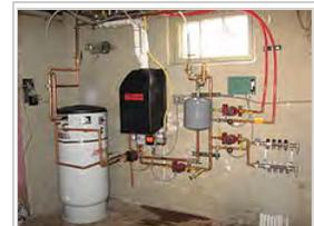
Gas-fired tankless condensing boiler with hot water storage tank (US)
