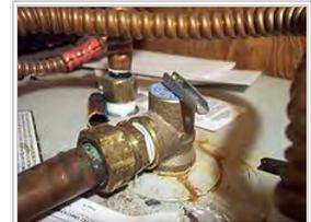
Temperature/pressure safety valve installed atop a tank-type water heater (US)
