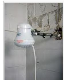
A poorly installed electric shower head can pose an electrical shock hazard
