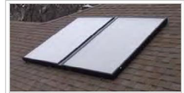
Flat-plate solar thermal collector, viewed from roof-level
