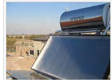
Roof-mounted close-coupled thermosiphon solar water heater.
