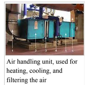
Air handling unit, used for heating, cooling, and filtering the air
