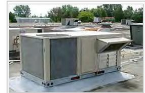
Rooftop HVAC unit with view of fresh air intake vent.
