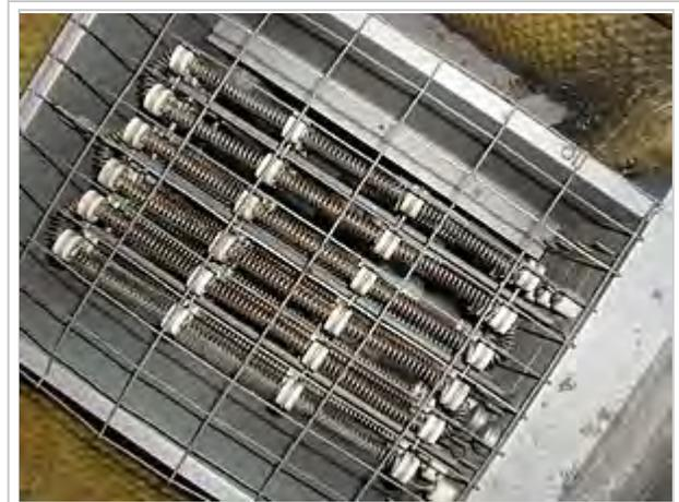
30 kW resistance heating coils
