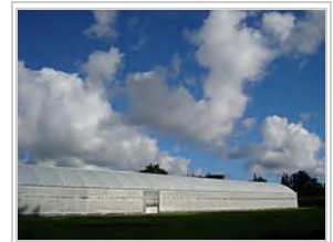
A plastic air-insulated greenhouse in New Zealand
