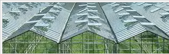
Greenhouses in the Westland region, Netherlands
