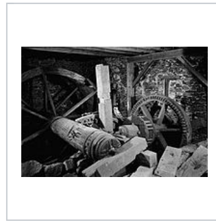
Gristmill drive machinery, Thomas Mill, Chester County, PA
