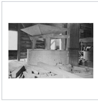
Gristmill hopper, Skyline Drive, VA, 1938. Grain was funneled through the hopper to a grinding stone below
