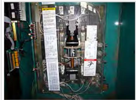
A Cummins Onan transfer switch
