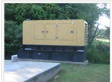
A 200 kW Caterpillar diesel generator set in a sound attenuated enclosure used as emergency backup at a sewage treatment substation in Atlanta, United States.
