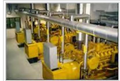
Internal combustion engines to generate electricity.<sup>[8]</sup>
