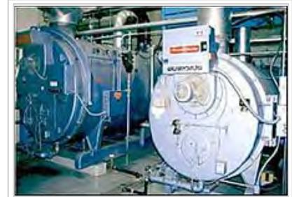
Boiler retrofitted to accept landfill gas.<sup>[8]</sup>
