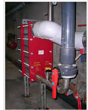
An interchangeable plate heat exchanger applied to the system of a swimming pool
