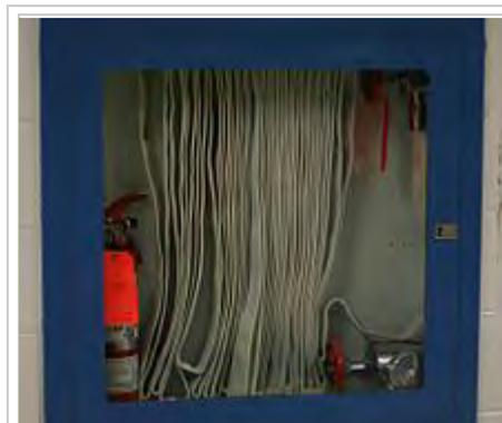
A fire safety station at a high school. Fire hoses built into a structure can sometimes be used by occupants to mitigate fires while the fire department is responding.
