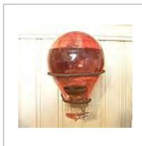
A glass grenade-style extinguisher, to be thrown into a fire.
