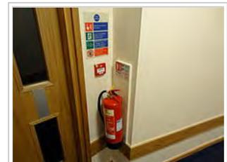
A British fire extinguisher with ID sign, call point and fire action sign
