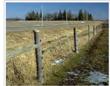
Electric fence of high tensile wire. Not all strands are electrified, only those attached to the fence posts with black insulators
