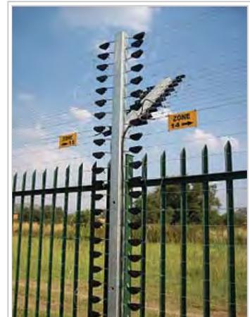
Multi-zone security electric fence used alongside a physical barrier.
