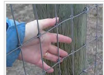
A closely spaced woven wire such as this "no climb" fence has a lower risk of animals becoming entrapped and injured. Note "knots" at each junction securing the wire together
