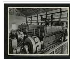
Three English Electric 7SRL diesel alternator sets being installed at the Saateni Power Station, Zanzibar 1955
