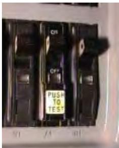
**The GFI circuit breaker** controls an entire circuit, and is installed as a replacement for a circuit breaker on your home's main circuit board. Some homes are wired so that all bathrooms or all outdoor fixtures are on the same circuit. Rather than install multiple GFI outlets, one GFI circuit breaker can protect the entire circuit.
