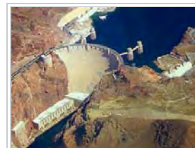
Large dams such as Hoover Dam can provide large amounts of hydroelectric power; it has 2.07 GW capability.
