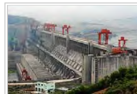
Large dams such as Three Gorges Dam in China can provide large amounts of hydroelectric power; it has a 22.5 GW capability.
