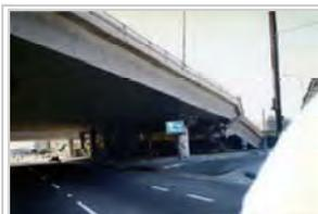
Insufficient shear reinforcement let main rebars to buckle, Northridge
