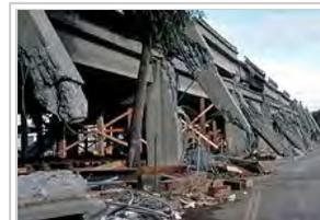
Support-columns and upper deck failure, Loma Prieta earthquake
