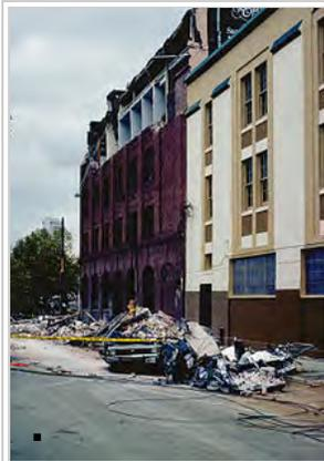
Typical damage to unreinforced masonry buildings at earthquakes
