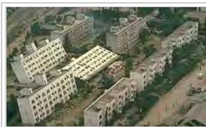
Effects of soil liquefaction during the 1964 Niigata earthquake
