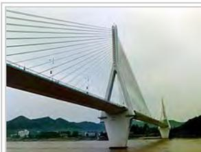
Prestressed concrete cable-stayed bridge over Yangtze river
