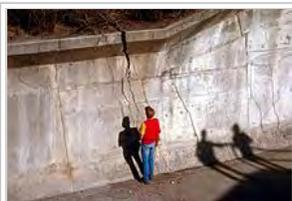
Failure of retaining wall due to ground movement, Loma Prieta
