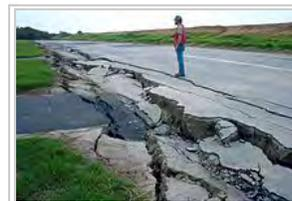
Lateral spreading mode of ground failure, Loma Prieta
