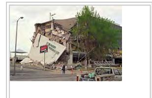
Effects of completely shattered joints of concrete frame, Northridge
