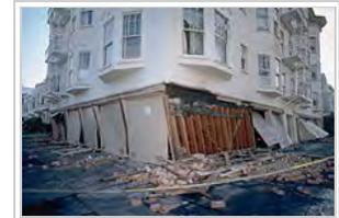
Soft story collapse due to inadequate shear strength at ground level, Loma Prieta earthquake
