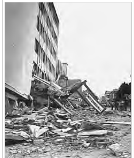
Collapsed Gran Hotel building in the San Salvador metropolis, after the shallow 1986 San Salvador earthquake.
