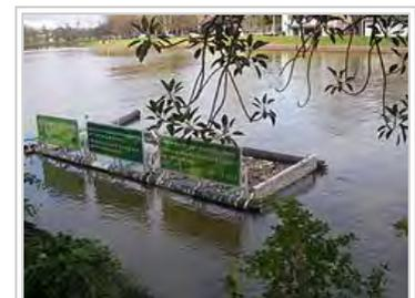
A litter trap catches floating waste in the Yarra River, east-central Victoria, Australia
