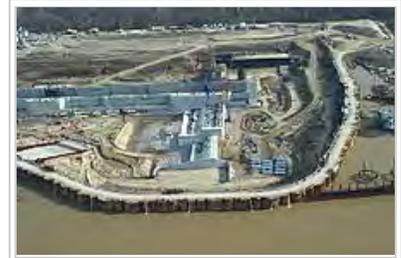
A cofferdam during the construction of locks at the Montgomery Point Lock and Dam
