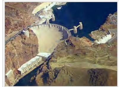
The Hoover Dam is an example of an arch-gravity dam.
