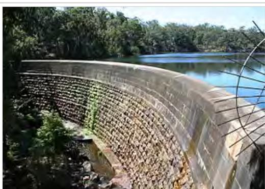
Masonry arch wall, Parramatta, New South Wales, the first engineered dam built in Australia
