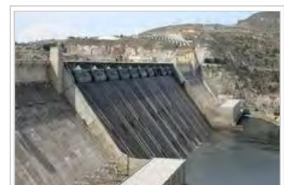
The Grand Coulee Dam is an example of a solid gravity dam.
