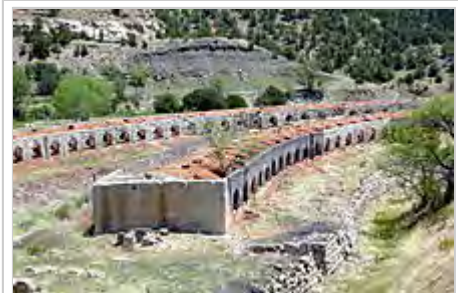
Coal coking ovens at Cokedale, west of Trinidad, Colorado, supplied steel mills in Pueblo, Colorado
