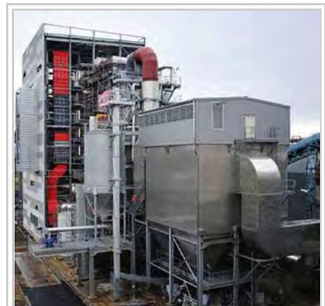
A cogeneration plant in Metz, France. The station uses waste wood biomass as an energy source, and provides electricity and heat for 30,000 dwellings.
