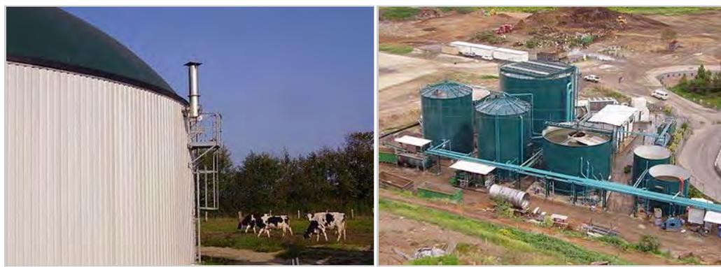
*Left:* Farm-based maize silage digester located near Neumünster in Germany, 2007 - the green, inflatable biogas holder is shown on top of the digester. *Right:* Two-stage, low solids, UASB digestion component of a mechanical biological treatment system near Tel Aviv; the process water is seen in balance tank and sequencing batch reactor, 2005.
