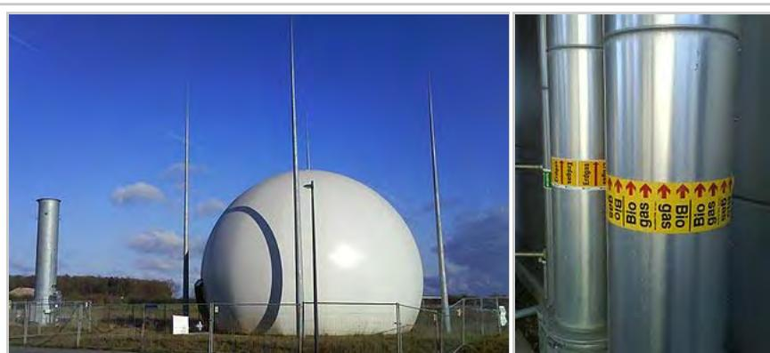
Biogas holder with lightning protection rods and backup gas flare      Biogas carrying pipes
