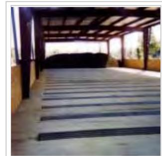
Channeled concrete floor of a composting pad for perforated piping that delivers oxygen to the composting mass
