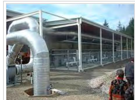
Aeration system for a closed chamber composting facility
