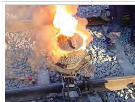
Thermite reaction proceeding for a railway welding. Shortly after this, the liquid iron flows into the mould around the rail gap
